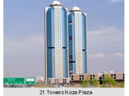
21 Towers Koza Plaza
